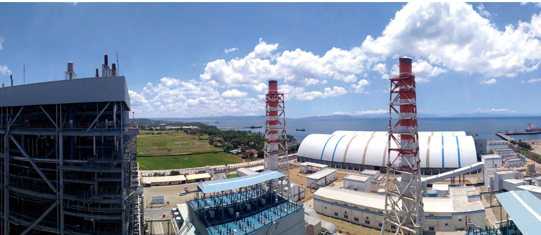
菲律宾普丁巴图 2X135MW 燃煤电站项目 The Project of Puting Bato 2X135MW Coal Power Plant in the Philippines
