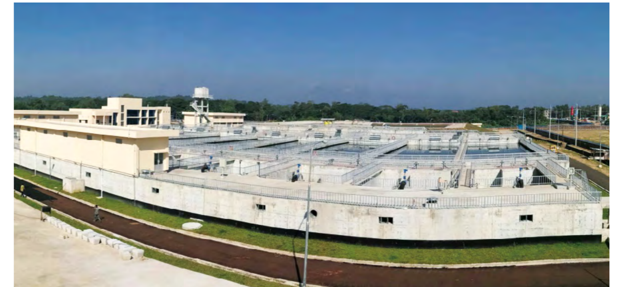
孟加拉哈西娜供水处理厂 The Hasina Water Supply Plant, Bangladesh
